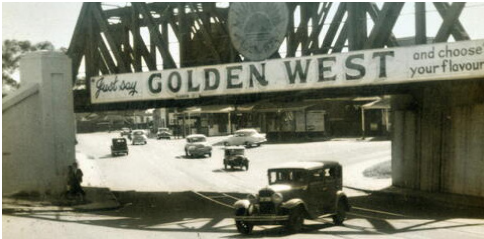
Cars driving on Guildford Road under the Mount Lawley Subway, travelling south towards the city, 1954. COV PH04226
