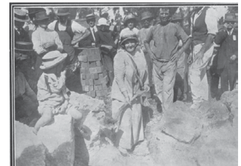
Digging the foundations for ANZAC Cottage, 1916. COV PH01006.
