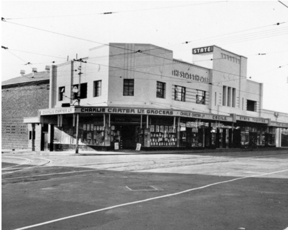
Lyceum Buildings, Mt. Lawley and the Lyceum Theatre, later the State Theatre and its art deco renovation, 1939 (SLWA)
