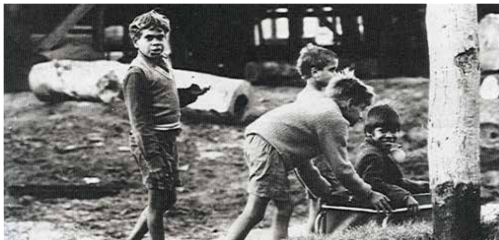
Image of Lindsay Calyun and friend in Miller's woodyard, early 1960s. Image from Powering Perth: A History of the East Perth Power Station space (2011), p 49.
