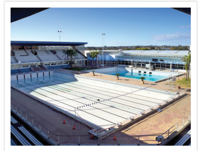
The main swimming pool after being drained, September 2011 (COV PH03949)
