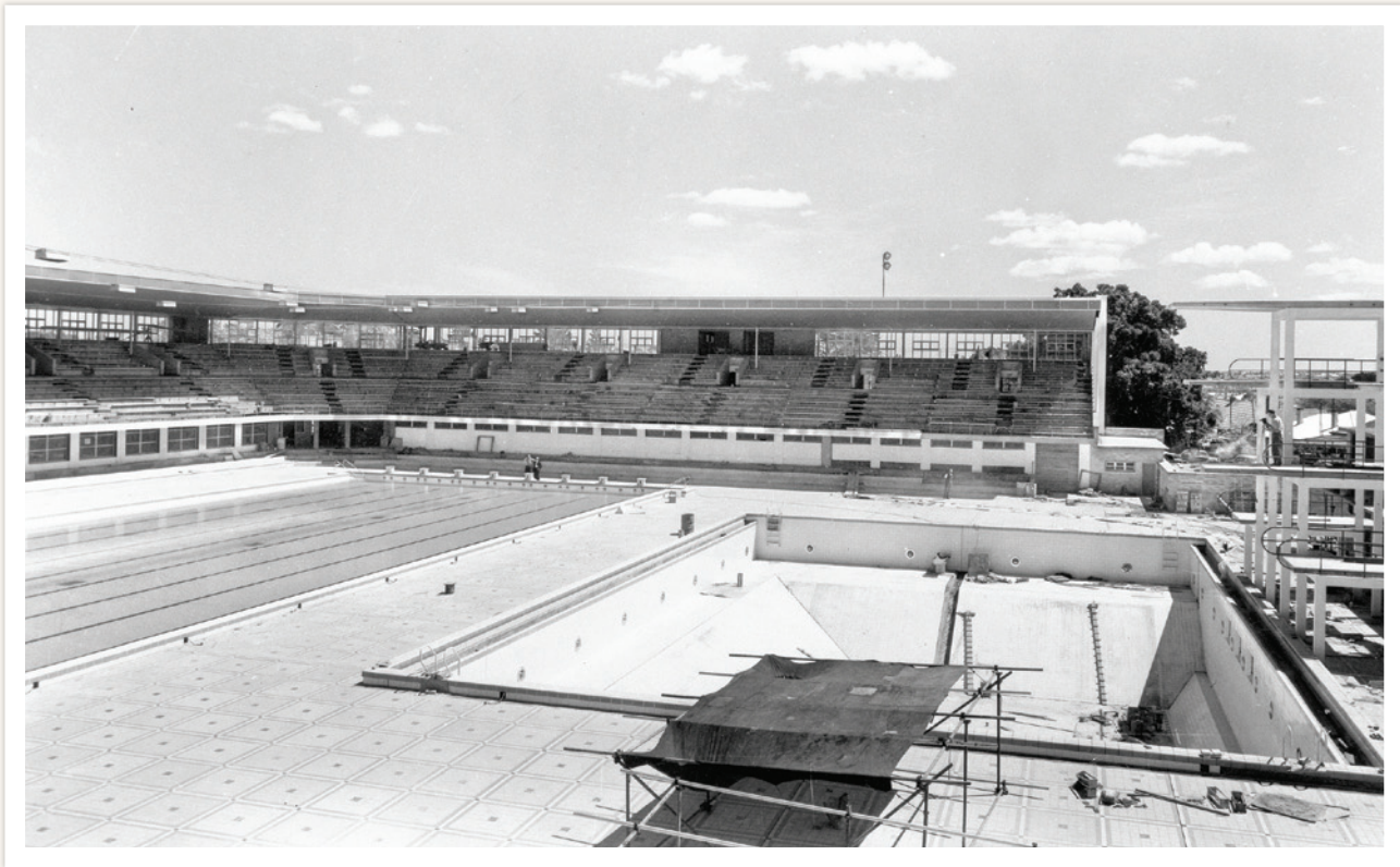
Tiling nearing completion, 30 September 1962 (COV PH0010)
